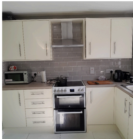
New kitchens in Ardilea Court & Snugville Street
