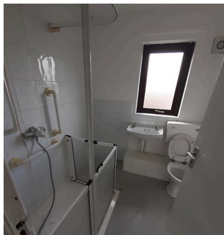
Bathroom before picture
