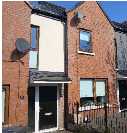
New canopies installed at Ardglan
