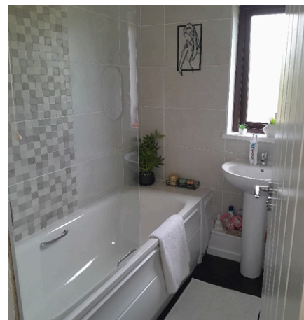
Bathrooms were installed at St Mary's Court & Flax Foyer
